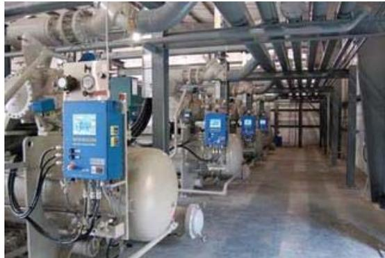
*Four Vilter compressors installed at the Shade Landfill in Somerset County. They increase the gas pressure to 200 psig (13.7 bar g) for processing by the Air Liquide system. Vilter has become an important supplier of LFG compressor equipment over the past two years*
