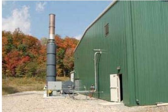
*The thermal oxidizer used to destroy the non-methane organic compounds that are removed from the LFG*
